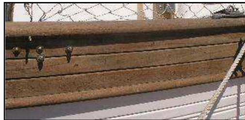
A close-up of our teak, about a month after applying a maintenance coat of Semco. Most of the other photos of ¿Qué Tal? show the Semco at a distance.
